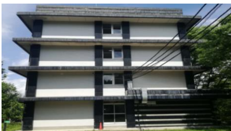
Fig. 9. Experiment with a four-floor building as target.
